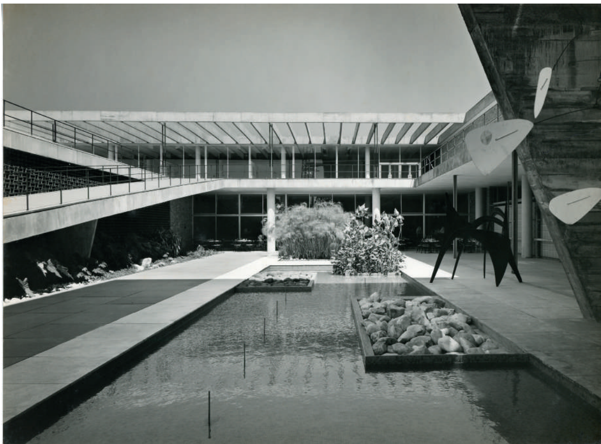
School building on the occasion of the Calder exhibition, 1959.
