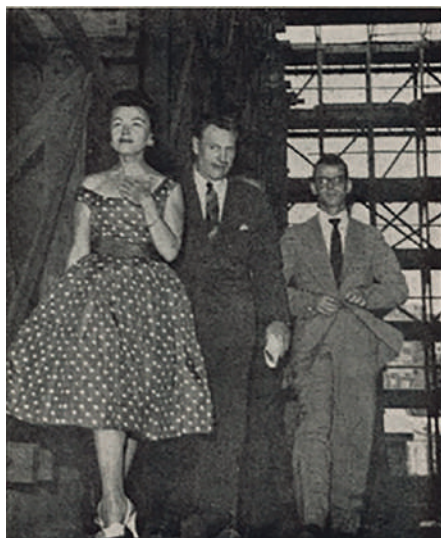
Fig. 59. Nelson Rockefeller, governor-elect of New York, visiting the construction site of MAM Rio, 1958, photograph. Source: Boletim do Museu de Arte Moderna do Rio de Janeiro , n. 17, January 1959, n. p. Collection: Research and Documentation MAM Rio.
