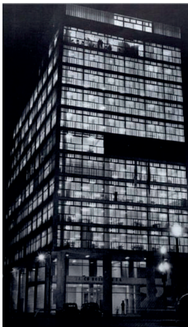
Fig. 2. Photograph of the Banco Boavista building on MAM Rio's inauguration in its new home on the 11th floor. Published in the February 1949 issue of Sombra magazine, in the article titled "The Museum of Modern Art."
